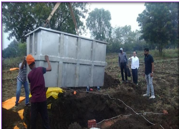
Plate 6: Installation of outer tank in pit
