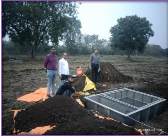
Plate 7: Installation of outer tank in pit
