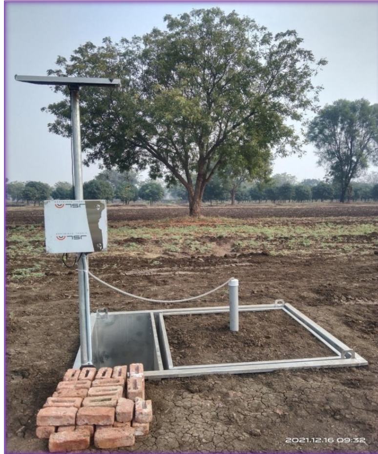
Plate 10: Installation of solar panel
