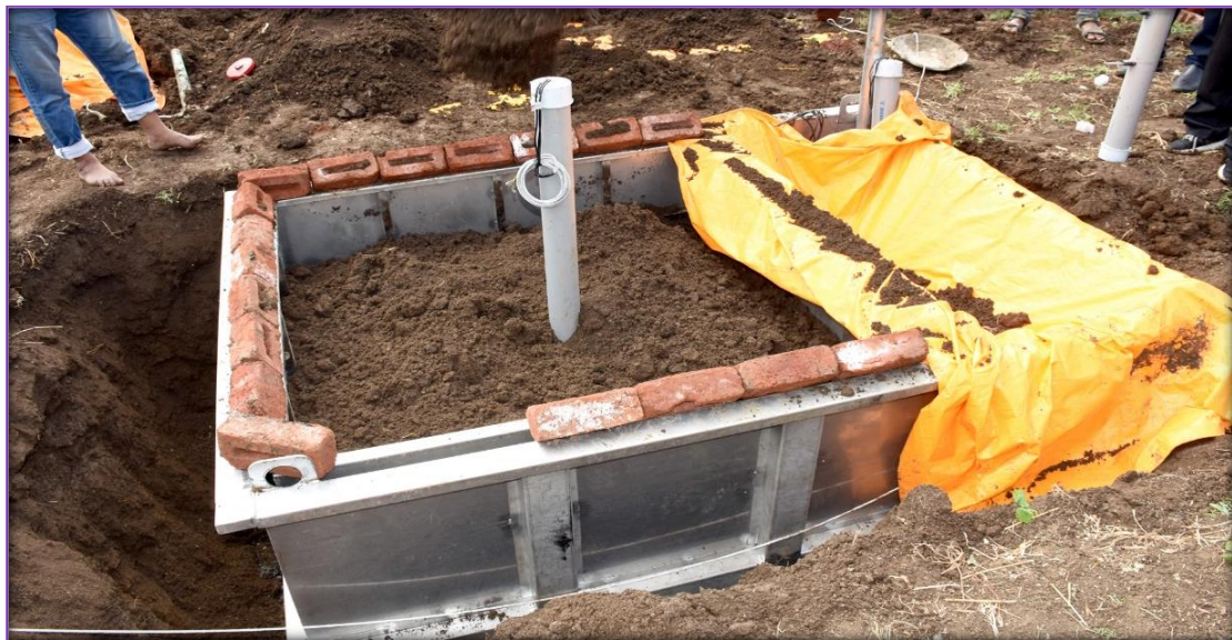
Plate 9: Installation of moisture and temperature sensor
