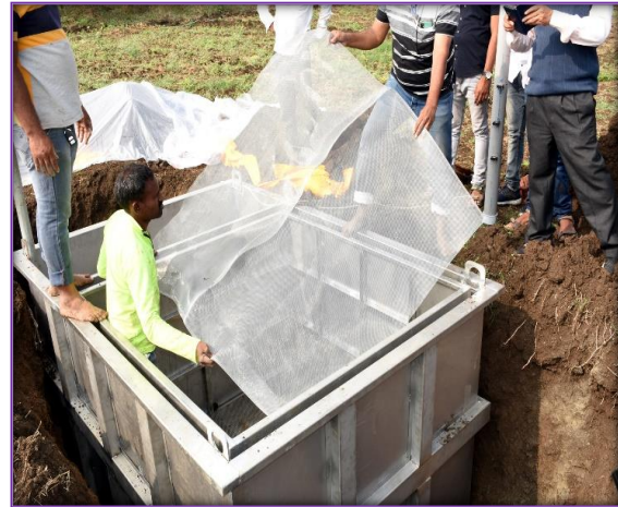
Plate 8: Steel net installation at bottom of inner tank
