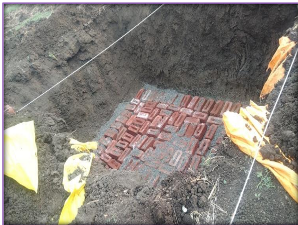
Plate 5: Sand and bricks layer laid at bottom of pit
